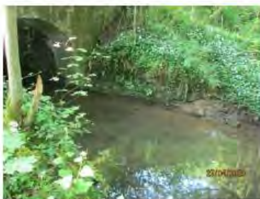
Amont de la station.
