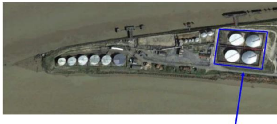
Cuvette 4- Stockage de Gazole
