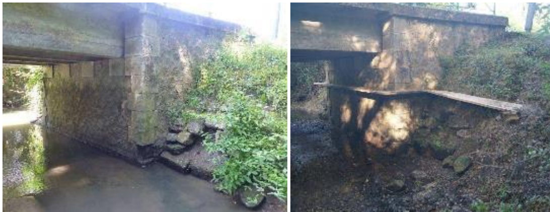
Figure 21 : Example of a layout for the ecological transparency of a structure by the installation of a corbelling (© CD33)
