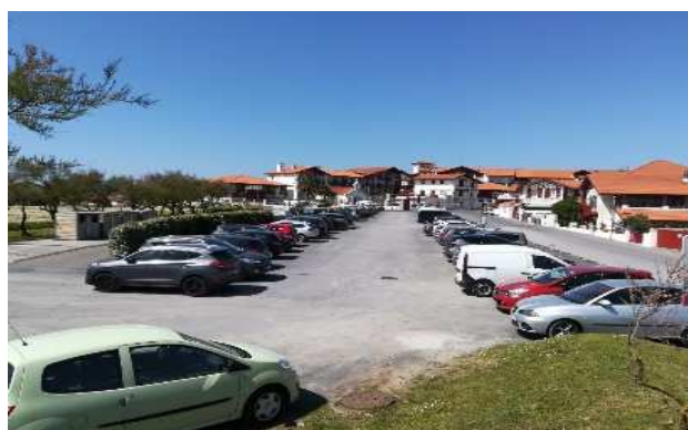
Bâtiments, routes, parking
