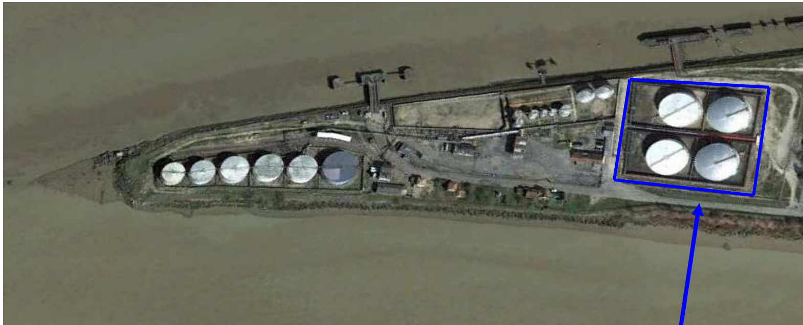
Cuvette 4- Stockage de Gazole
