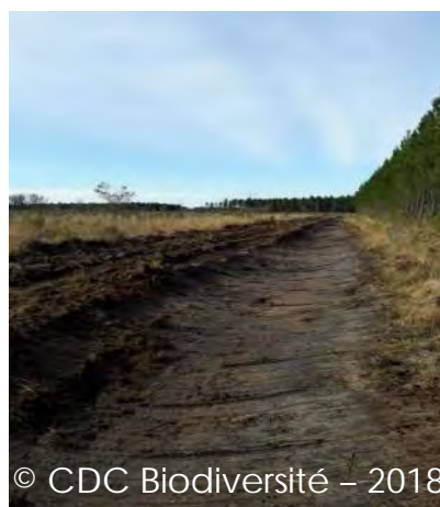
Figure 140 : Fossés reprofilés – image post-travaux
