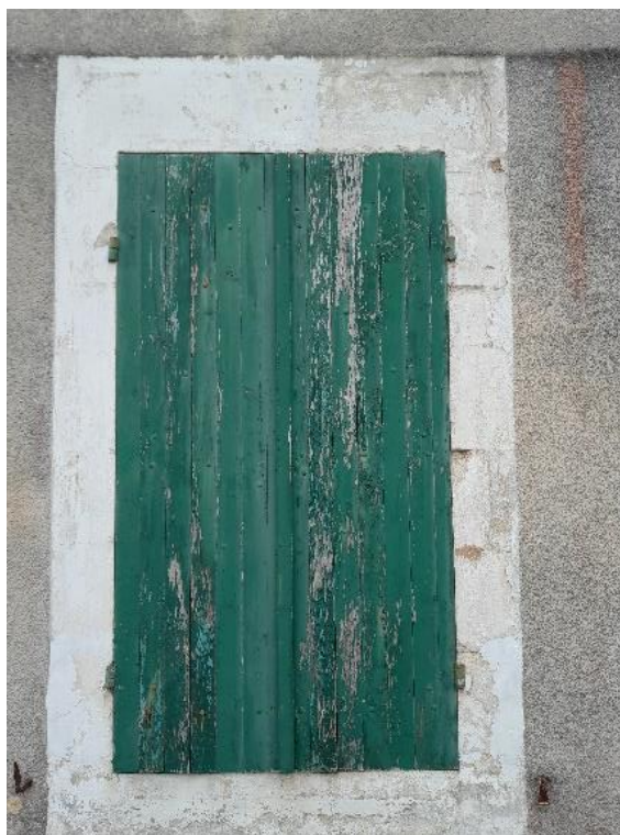
Photo 17: Volet façade Sud
