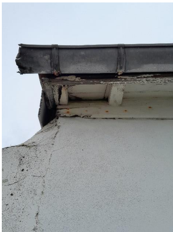
Photo 11: Angle façade Sud
