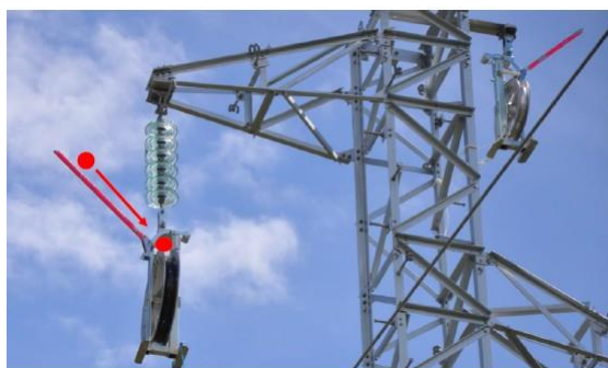
Figure 21 : installation des poulies
