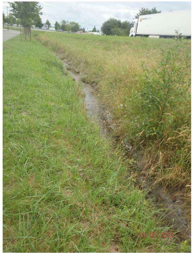
Photo 5 – Fossé pluvial bordure A64/Eurolacq 2 direction péage
